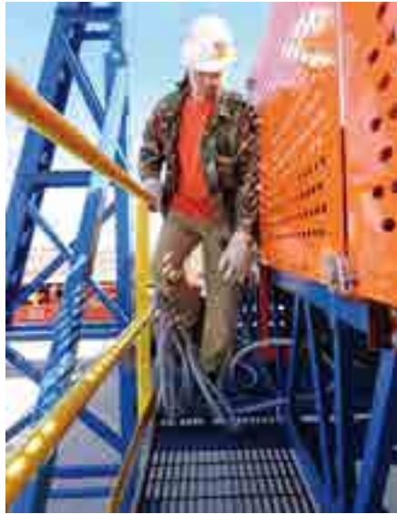
OBSTRUCTIONS SUCH AS DISCARDED COMPONENTS, TOOLS OR SPILLAGE CAN CAUSE A SLIP, TRIP OR FALL INJURY © MARTIN ENGINEERING 2021
