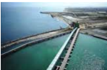
View from the pier: the last section of the Pipe Conveyor runs along the sea to the transfer tower.
