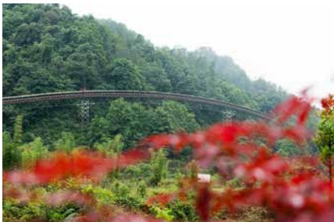
*Whenever technically possible, the routing of the conveyor has been adapted to the topography.
