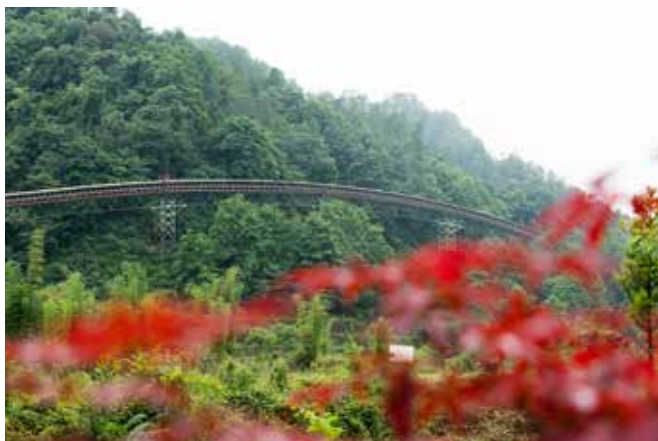
Whenever technically possible, the routing of the conveyor has been adapted to the topography. Photo credits: BEUMER Group GmbH & Co. KG
