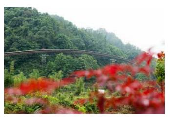
Whenever technically possible, the routing of the conveyor has been adapted to the topography. Photo credits: BEUMER Group GmbH & Co. KG
